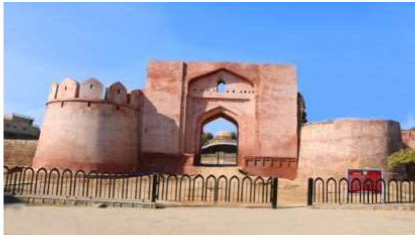
Fig 2. Façade of Rewat Fort
