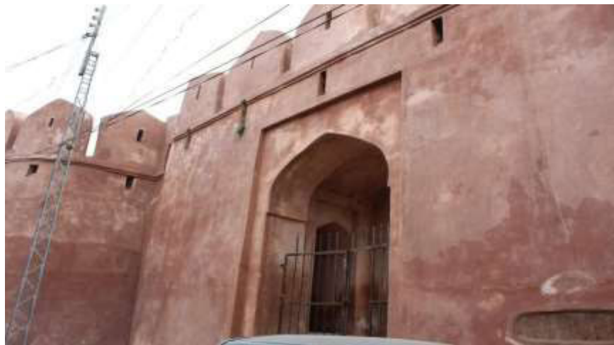
Fig.17. Northern gate and Bastion of the Fort (view from outer side)
