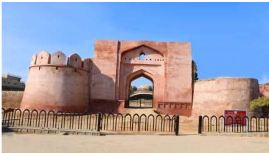
Fig.16. Façade of Rewat Fort
