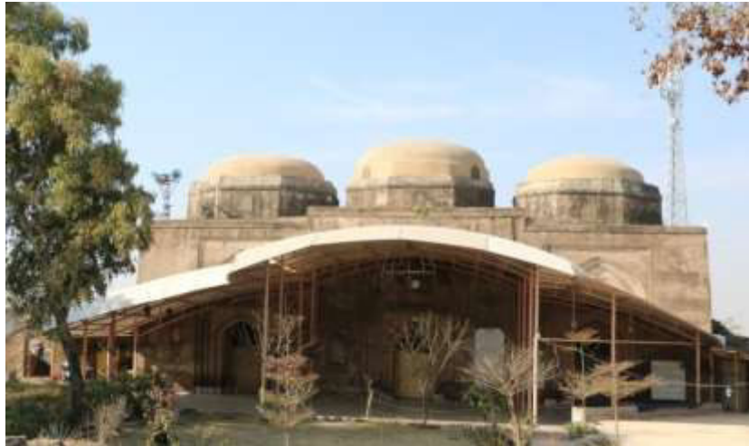
Fig 4. The Mosque of Rewat Fort.
