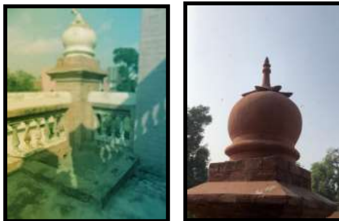
Figure 35: condition of cupola in 2016 v/s 2021 Source: author
