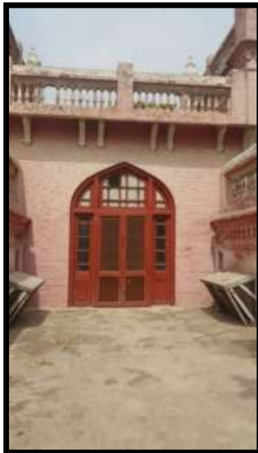
Figure 15: Original floor at the terrace Source: author
