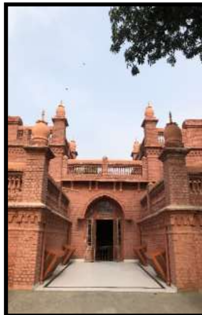
Figure 16: Present condition of the terrace Source: author
